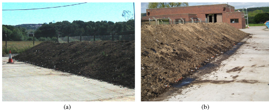
Fig. 6. Windrow trial, showing (a) increased settlement at crest and (b) increased drainage at the base.
